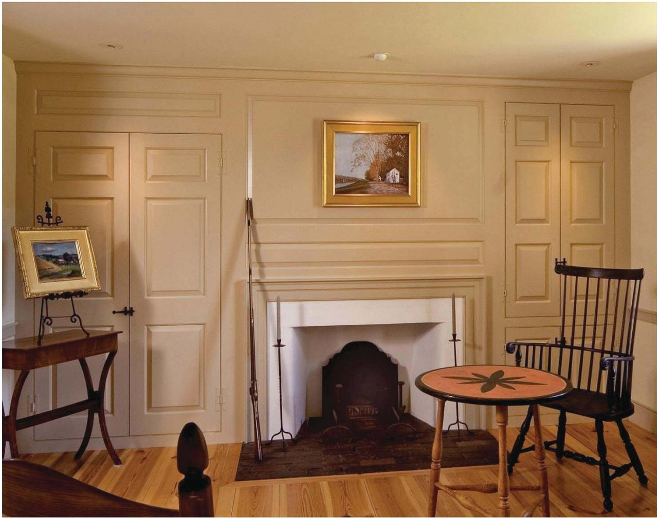
**PANELING** Wood raised paneling and beaded paneling for home interiors. The paneling above was installed in a stone farmhouse in Solebury, PA. It was designed to replicate the original paneling that was removed during a prior renovation.
